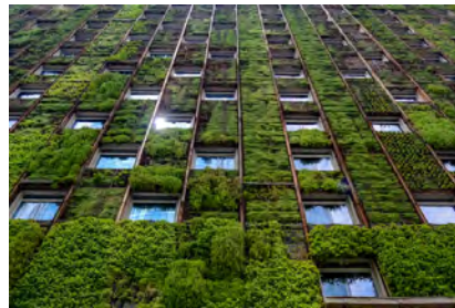
An example of a green wall
