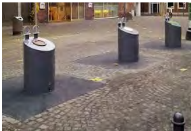
An example of underground waste storage
